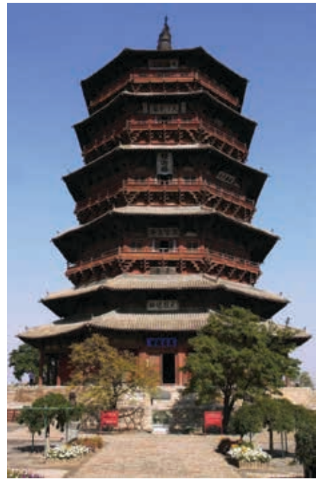
The 67 m high, nine-storey wooden pagoda of Yingxian County in Shanxi Province, China, completed in 1056, is one of the world's oldest standing multi-storey wooden structures
