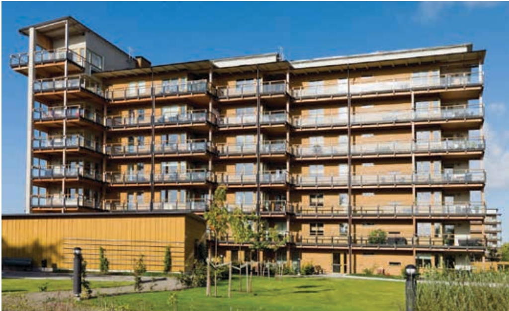
Eight-storey wood-frame low-energy apartment building constructed in 2009 using CLT structural system, Växjö, Sweden
